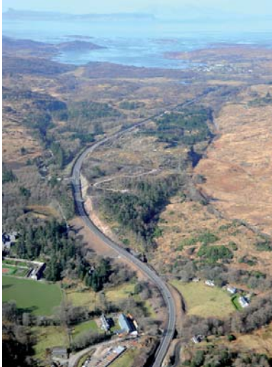
The Route West of Borrodale
