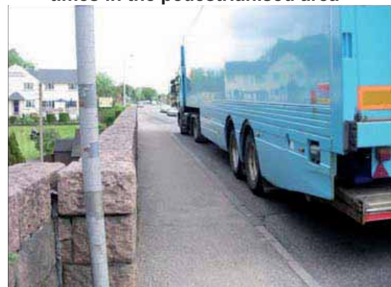
Figure 3-11: Physical restrictions on Belford Road/A82 will make providing for cyclists and pedestrians problematic
