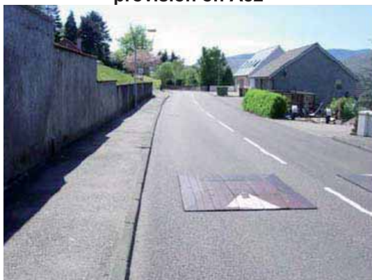
Figure 3-10: a number of streets in the old part of town benefit from traffic calming
