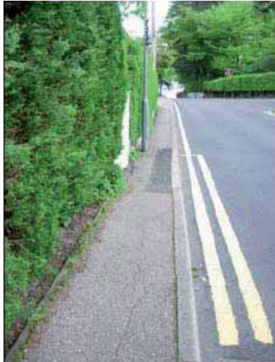
Figure 3-6: Typical narrow footway in older parts of Fort William
