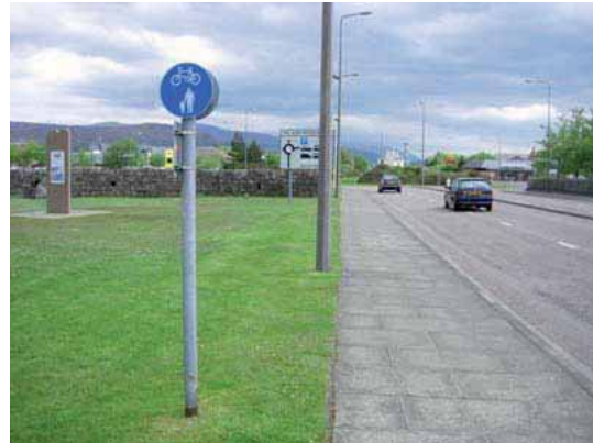
Figure 3-19: Poor designation of footway/cycle track at the old fort
