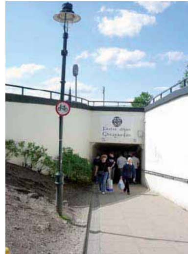
Figure 3-13: The underpass to the town is unattractive
