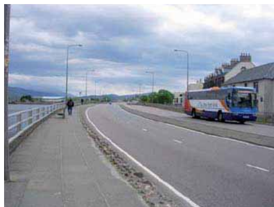
Figure 3-15: The footway and carriageway along the waterfront are underutilised
