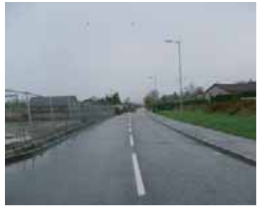
3a Investigative work is required on Obsdale Road to determine most suitable type of facility for cyclists.
