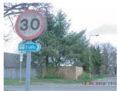
2c Signage is ambiguous at junction of Novar Road/B817.
