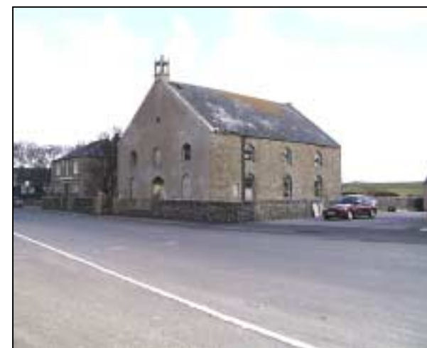
Below - former church with potential for conversion to business community or residential use.
