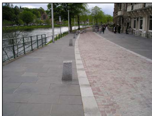
Figure 3.9.1: High Amenity Paving
