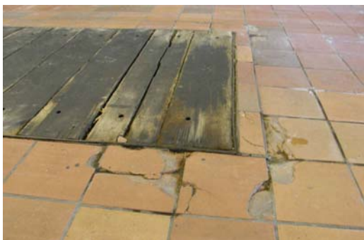
02 – Inspection pit in appliance bays
