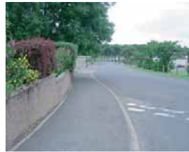
2f Flush dropped crossings and tactile paving are needed on Millbank Road, especially near the swimming pool.
