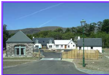
Rented housing in Applecross provided by Albyn Housing Society on land provided by The Highlands Small Communities Housing Trust.
