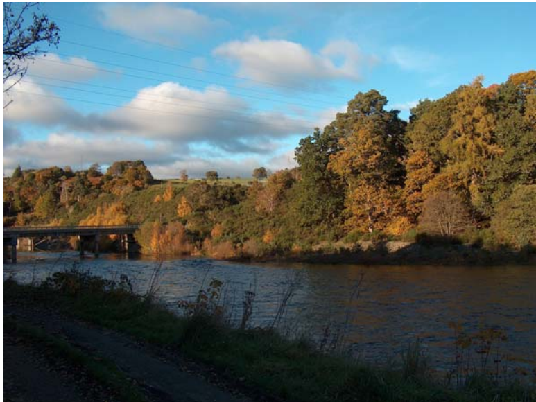
Figure A8.3: East of bridge over Beaulieu looking north
