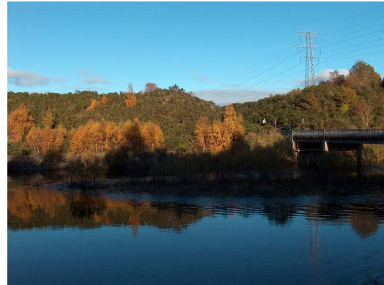
Figure A8.2: West of bridge over Beaulieu looking north west
