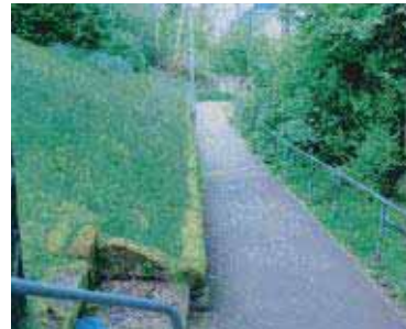
6b Parts of these well used steps to the town centre are not overlooked and may benefit from installation of CCTV.
