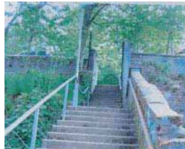
6a Handrail provision is good for each set of steps.
