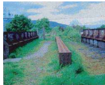
7b The bridge over the railway is still in place.
