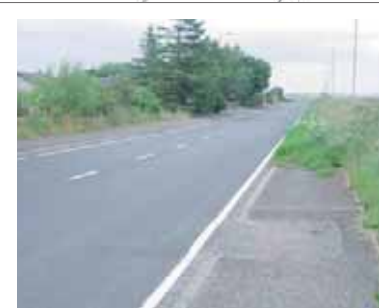
4c A shared use footway/cycle track is required on the A836 to the business park.
