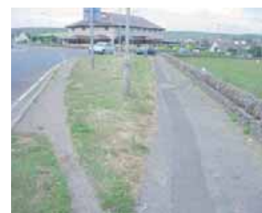
4a The pedestrian facilities at the junction of the A9 and A836 do not serve pedestrian desire lines.
