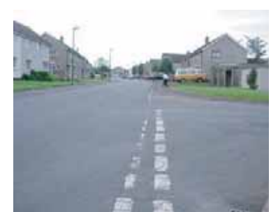
5b Junction mouths on Castlegreen Road could be reduced in width to aid pedestrians. Further investigation is needed to determine how this local distributor road can be made more cycle friendly.
