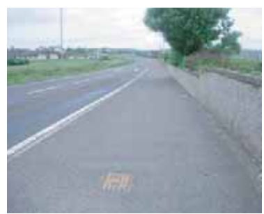
4a The footway on Scrabster Road could be easily converted to shared use for cyclists and pedestrians.
