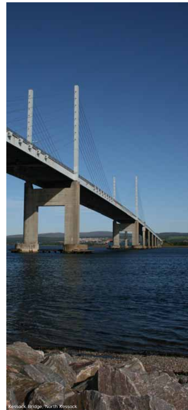
Kessock Bridge, North Kessock
