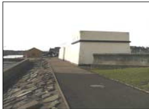
Photo: existing sewage macerator at Thurso
