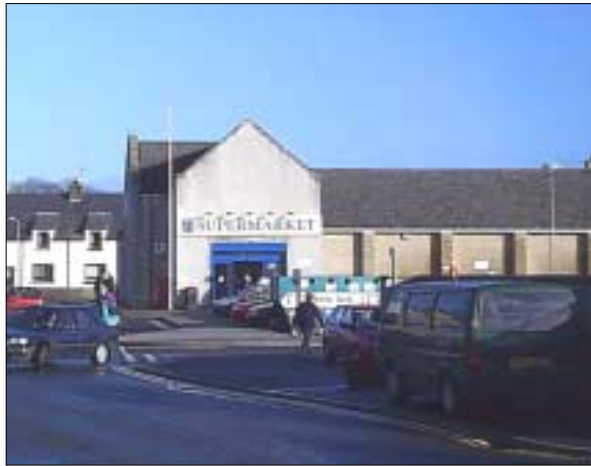
Photo: Town centre redevelopment
