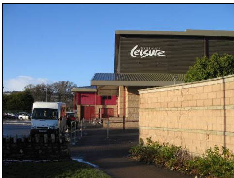
Figure 11 – Pedestrian provision at the Inverness Leisure site.
