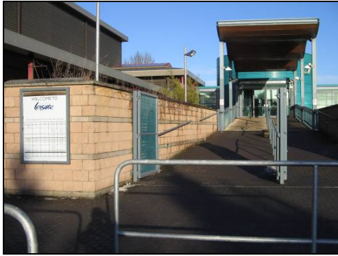
Figure 13 – Sloped access up to the main entrance.
