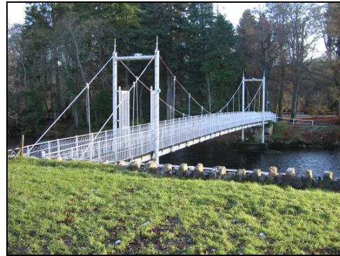
Figure 10 – A pedestrian foot bridge forming part of a pedestrian route across the River Ness close to Inverness Leisure.
