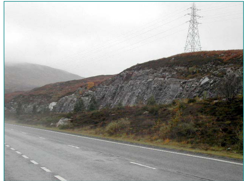
Figure A9.4: South of Drumochter Pass - Existing 132kV circuits
