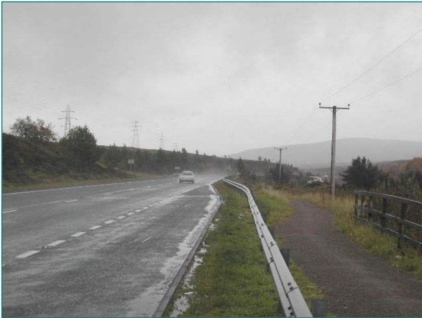
Figure A9.3: South of Drumochter Pass looking south
