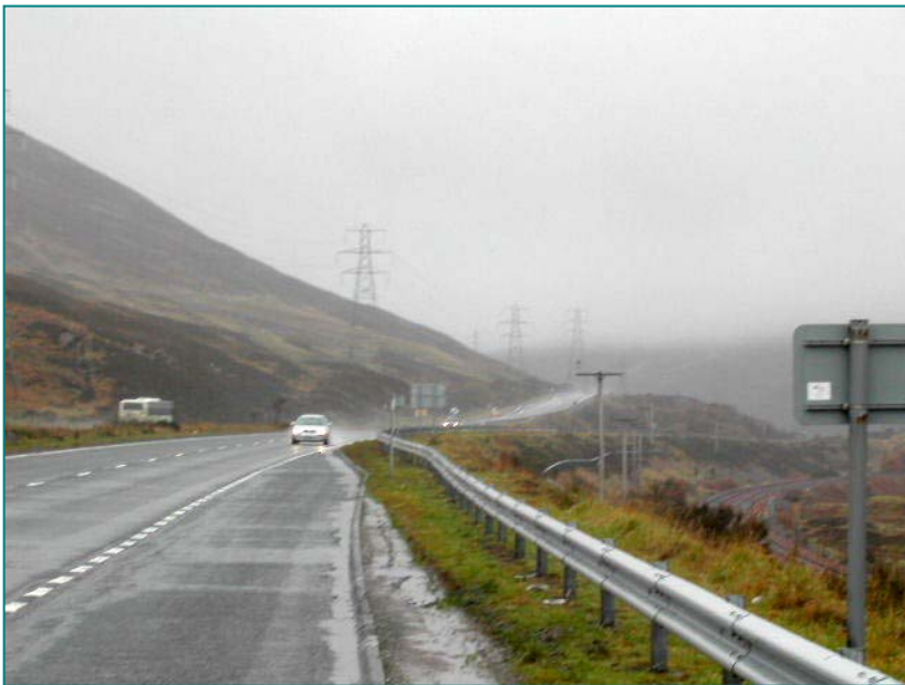
Figure A9.7: A9 Dual carriageway south of Drumochter looking south
