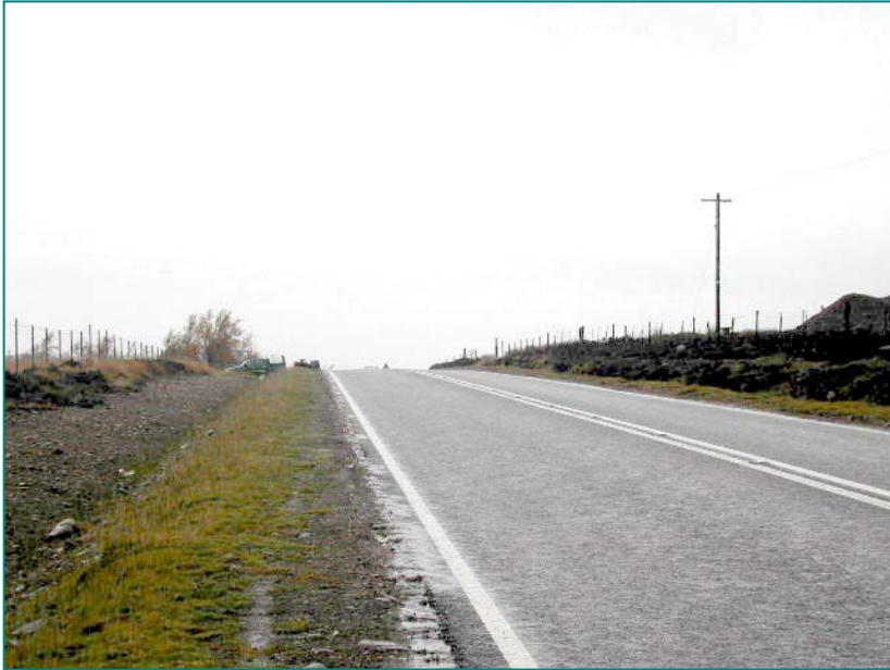
Figure A9.14: A889 north of Dalwhinnie looking north
