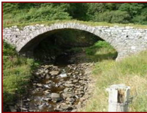
Category C(s) listed bridge over burn at Latheronwheel harbour
