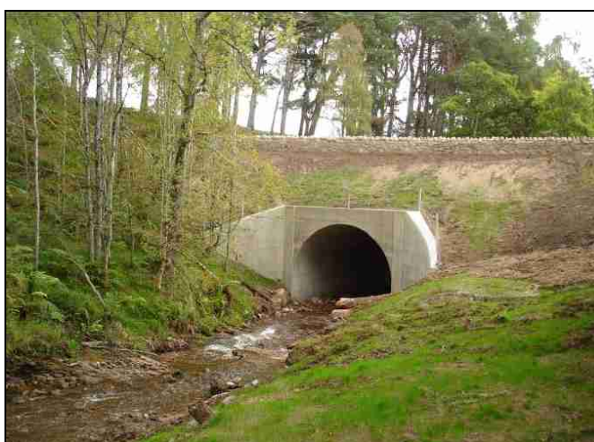
Figure 8.2: Quebec Bridge Replacement Completed
