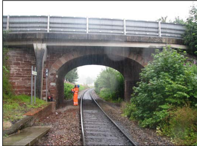
Figure 3.8.1: Bridge Inspection: Road Over Rail
