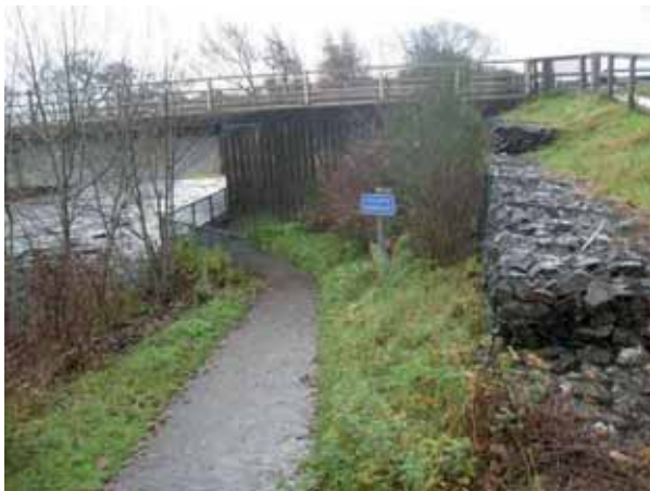
Figure 5-7: Sign instructing cyclists to dismount due to low overhead clearance and poor sightlines at underpass of A9.
