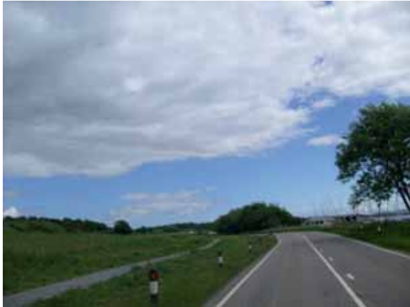
Figure 3-17: New footway on northern verge of B817
