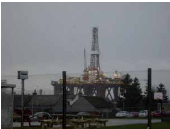
Figure 3-8: Oil rig at Invergordon Port
