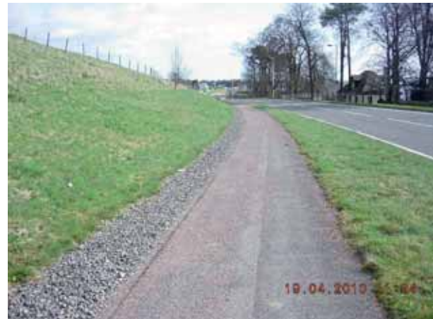
Figure 5-2: Existing footway between Alness and Belle Port
