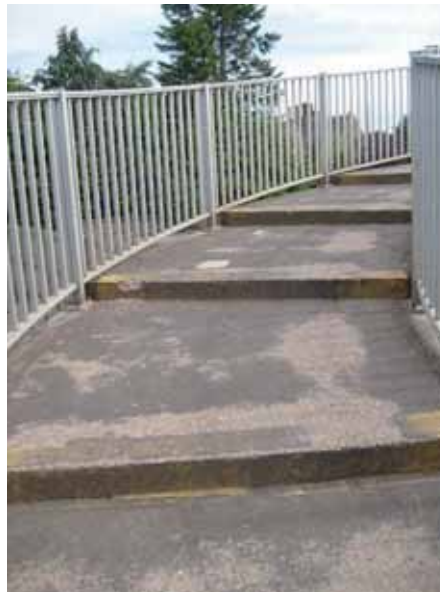
Figure 3-23: Stepped bridge over railway in Alness
