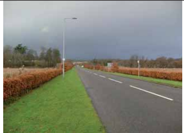
Figure 3-7: No pedestrian facilities on road linking A9 and B817.
