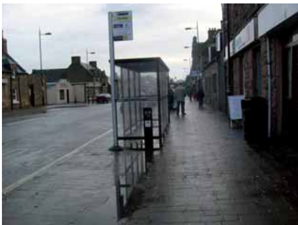
Figure 5-12: Bus shelter in Alness with flag and pole with timetable information attached. No seat or resting area in bus shelter.
