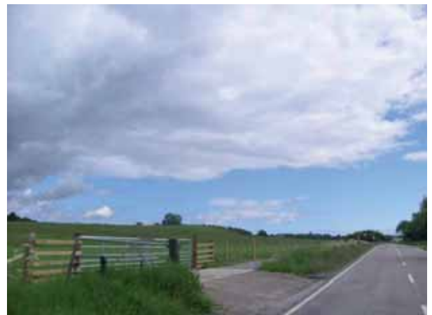
Figure 3-16: New footway on northern verge of B817
