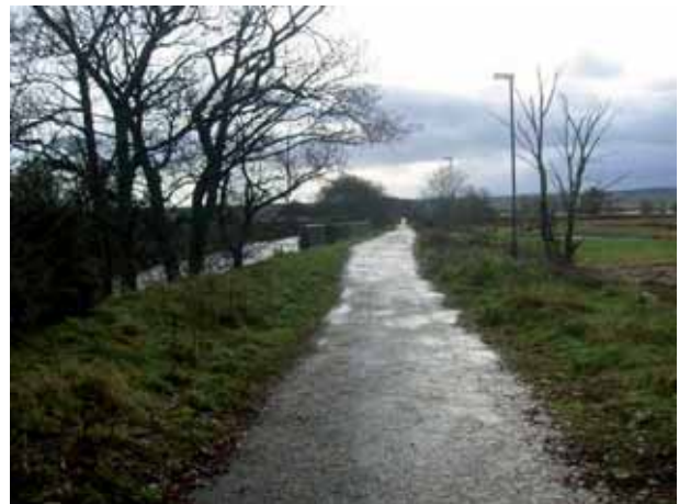
Figure 5-6: Section of riverside cycle route with excellent surface quality and lighting.
