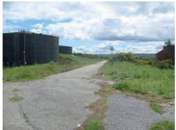
Figure 3-13: Informal path through Seabank Tank Farm
