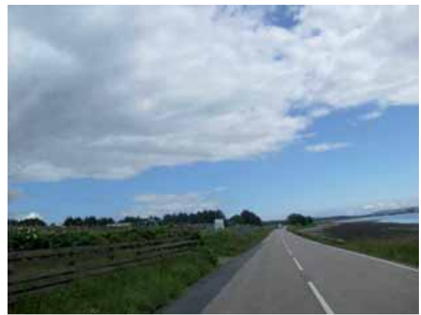
Figure 5-4: Pinch point as retaining wall on either side of the carriageway results in limited space for pedestrians and cyclists
