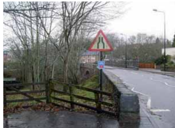
Figure 3-27: NCN Route 1 on-road signage on Alness High Street at Alness Bridge
