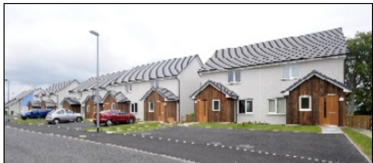
New tenant Ashleigh Rae is pictured (left) with Alex Neil, Scotland's Minister for Housing and Communities. The new housing at Knocknagael, Slackbuie is pictured above.
