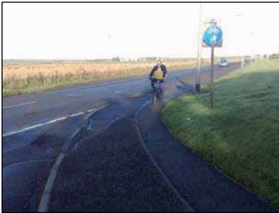
Figure 3-10: Shared use path along A99 North Road
