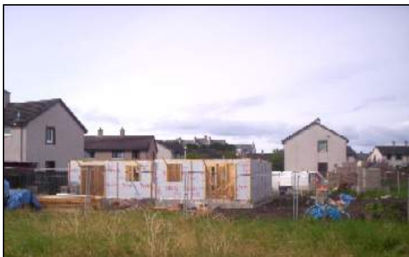
'GRO Grant' houses under construction at Elizabeth Crescent, Dornoch
