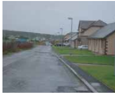
4k Inadequate footway in new build areas.
