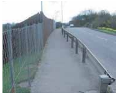
5a Footway narrows on approach to supermarket in Alness on railway bridge.
