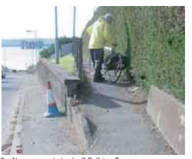
6e Narrow ramp to track off Golfview Terrace.
