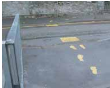
4j Crossing point at Perrins Road - a zebra crossing may be more appropriate.
