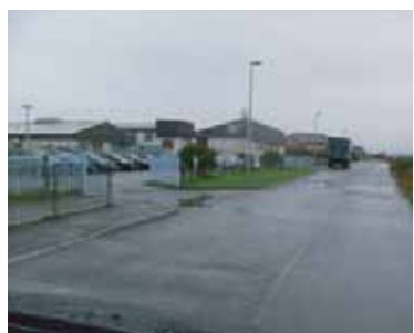
4k Section of footway missing from Obsdale Primary School.
