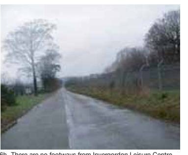
6h There are no footways from Invergordon Leisure Centre towards the industrial estates.
