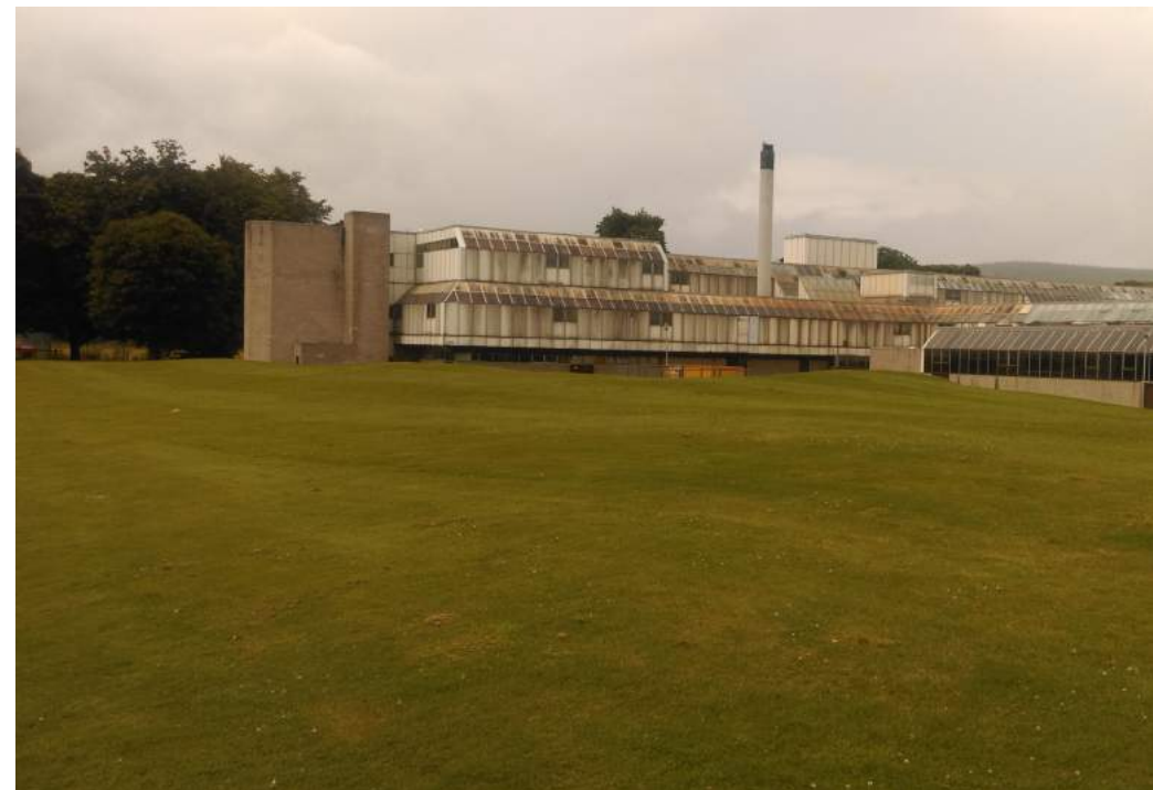
VIEW TOWARDS REAR OF ACADEMY BUILDING
