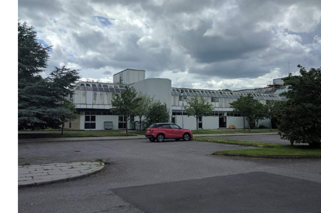
VIEW TOWARDS MAIN ENTRANCE
