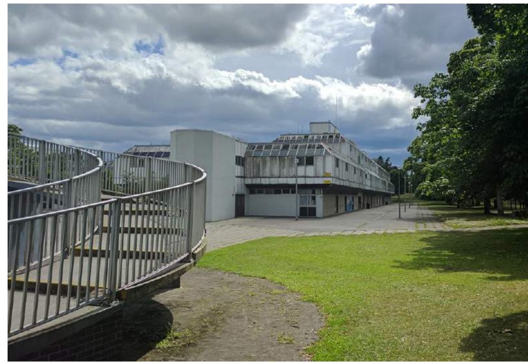
VIEW OF EXISTING BUILDING
