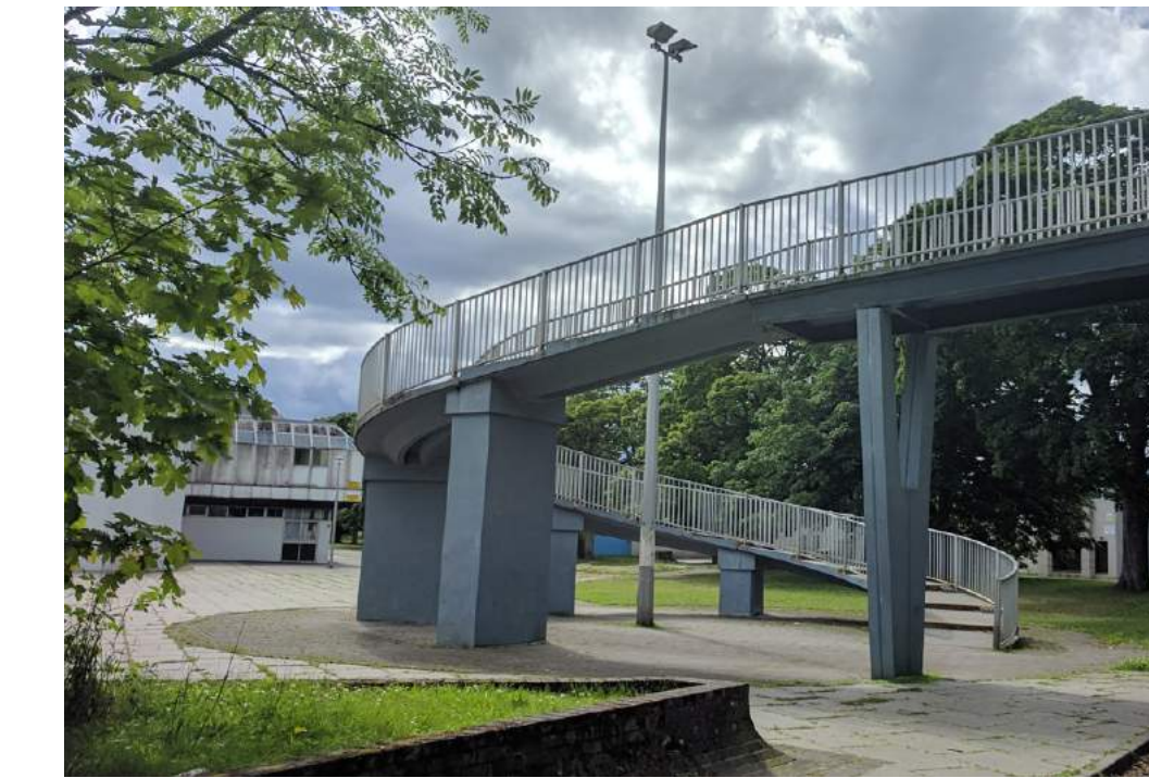
VIEW FROM PEDESTRIAN BRIDGE
