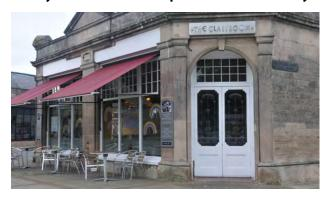
The blinds provide shelter for external tables and are retracted into unobtrusive purpose-built blind boxes under the fascia.
