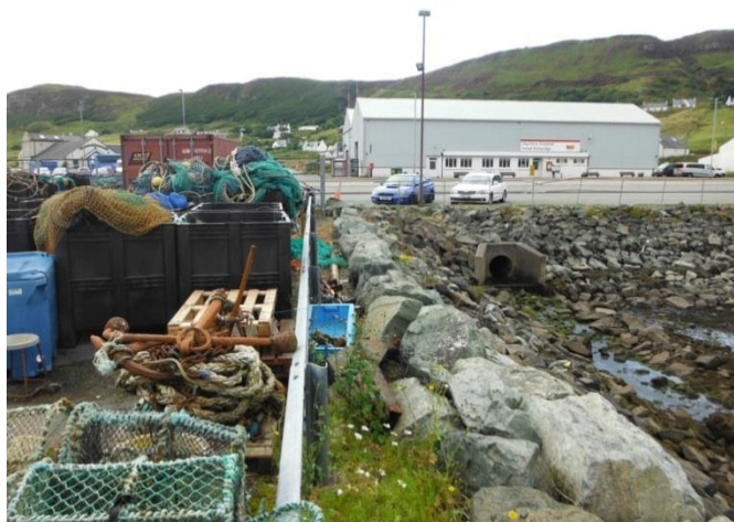
Photograph 9-2 Culvert Overflow of Small Watercourse
