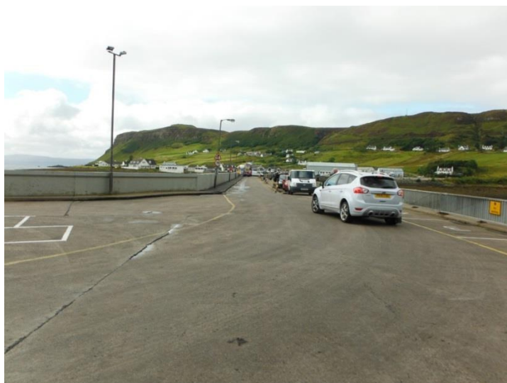
Photograph 9-1 Wall Protecting Pedestrians Along the Pier
