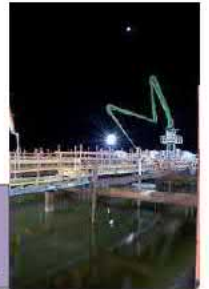
CONCRETE Concrete approachway widened from barge or end-over construction.
