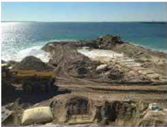
RECLAMATION Land reclamation by compaction of layers of granular material.
