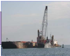
DREDGING Dredging by off-shore floating plant and disposal via barge.
