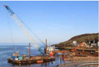
ROCK ARMOURING Rock armour placement around perimeter of land reclamation.
