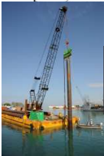
PILING Tubular piles and/or sheet piling driven from barge or over end construction.
