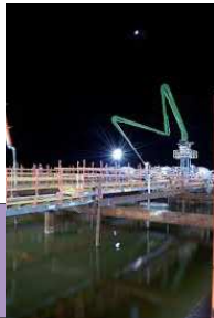
CONCRETE Concrete approachway widened from barge or end-over construction.
