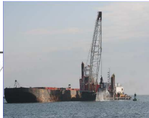
DREDGING Dredging by off-shore floating plant and disposal via barge.
