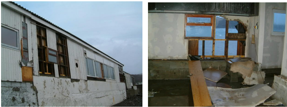
Figure 5-17. Damage to properties caused by the storm on 11 th -12 th January 2005
