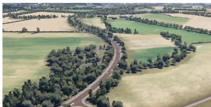
Looking south across scheme from A96 Smithton Junction
