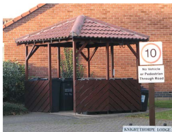
Good example of communal bin storage area
