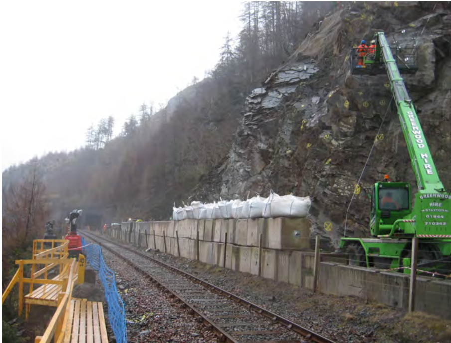
Figure 4.7 Temporary Rock Protection April 2012
