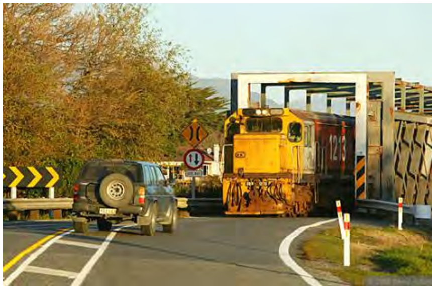
Figure 4.4 – Shared Road and Railway Bridge, New Zealand
