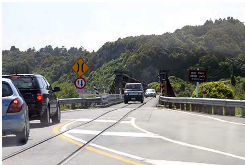
Figure 4.5 – Shared Road and Railway Bridge, New Zealand
