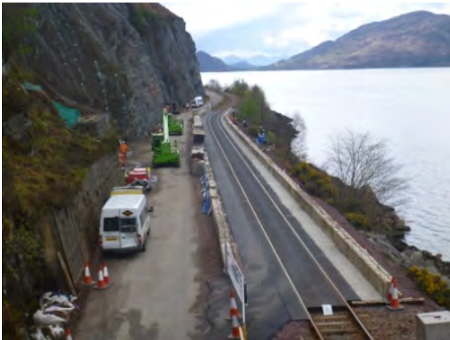
Figure 4.3 Temporay Road Diversion April 2012
