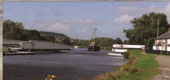
The new swing bridge will allow the canal to be operated anytime during the day. Currently there is a restriction during the morning and evening rush hours.
