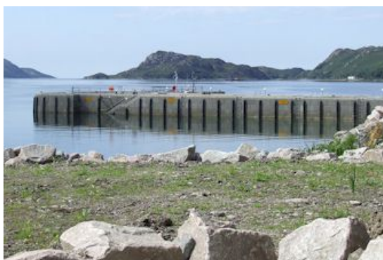
Photo 3 - The new pier at Inverie
