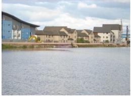
Patterned concrete walls with pigment have been completed on the riverside section of work. The stone cladding to the concrete walls have now started and it is hoped to have this completed by the end of this month. Backfilling to the wall and a stone cope to finish the wall will be completed shortly after this.
