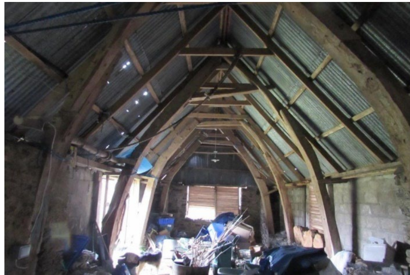
Fernaig cruck-framed barn, B-listed
