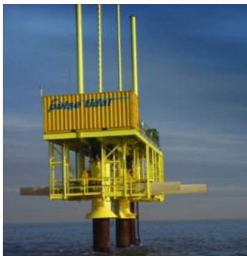
Figure 5 Pulse Stream 100 (0.1MW) TSD
