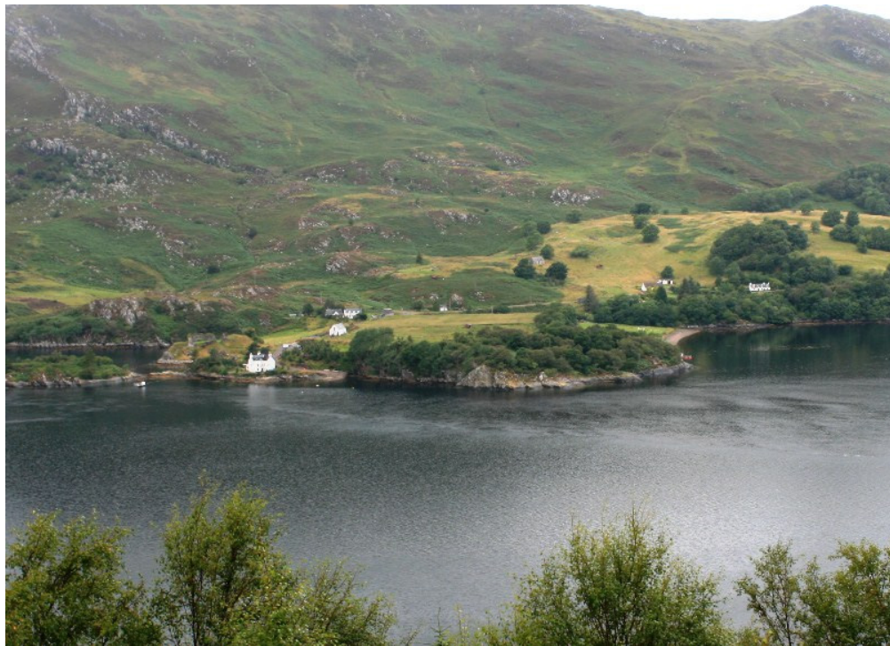
Photograph 1: Looking North across the Narrows from Strome Ferry. The spit of land would provide an ideal position for the approach to any tunnel or bridge option; however the existing dwellings and the Castle may cause planning concerns.
