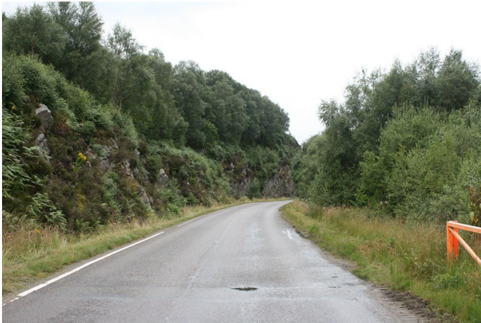
Photograph 9: Approach to possible Northern Portal position (facing south west). It may be advisable to straighten the road leading to the portal by realigning the bend through the removal of the free face at the left hand side of the bend.
