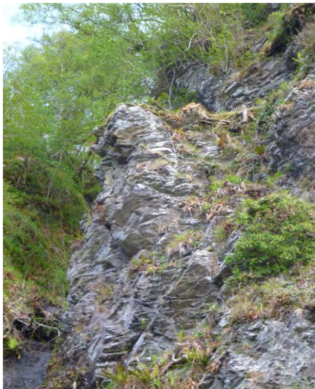
Photo 2: AA8 - 30m 3 pinnacle previously subjected to root jacking.
