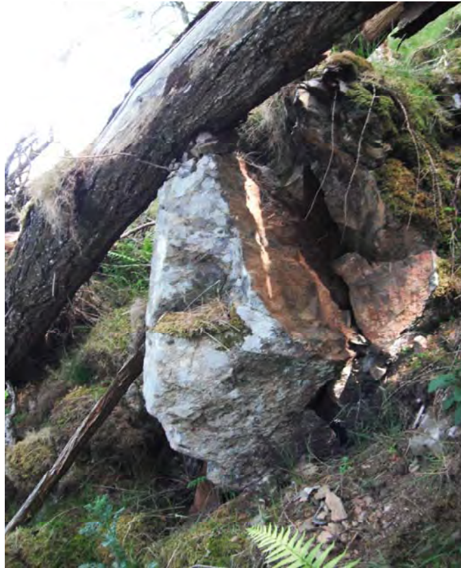
Photo 7: AA16-17 Upper - Unstable detached blocks retained only by fallen trees.
