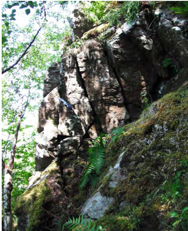
Photo 8: AA16-17 Upper 5 No. block ( 0.6\text{m}^3 each) prone to toppling.
