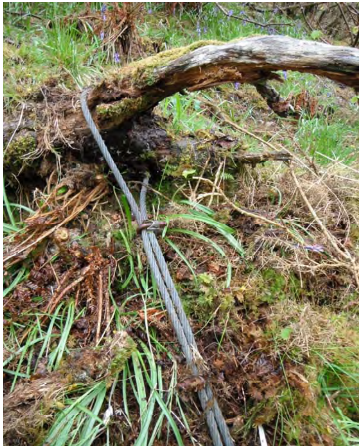
Photo 4: AA14W - Top cable anchor consisting of a rotting tree stump.
