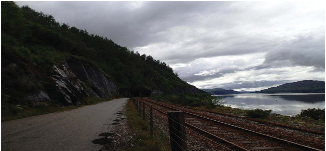
Photograph E06 – Online Corridor looking towards the Avalanche Shelter
