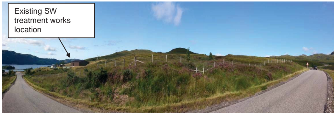
Photograph P02 – Scottish Water treatment plant (to the left) and looking north along A896 where the N9 alignment will join (to the right).
