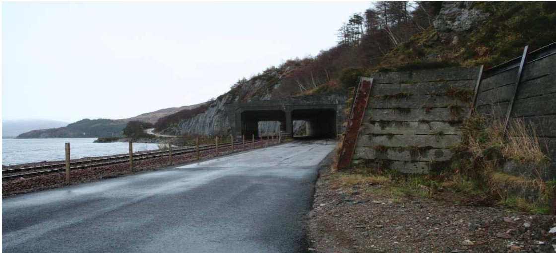
Photograph P10 – Existing A890 looking north-east toward the avalanche shelter
