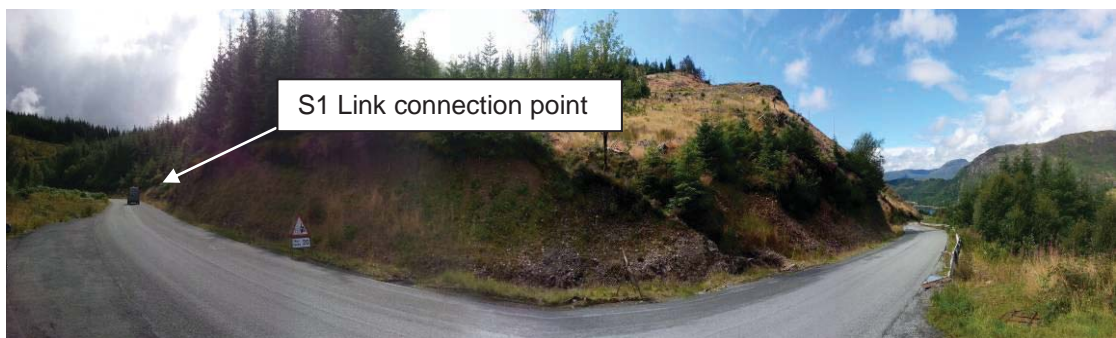
Photograph P07 – S1 Link Road at A890 connection point
