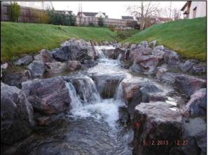
The works involved shoring up of the affected area and the introduction of a series of step pools which allow the water to cascade down the steep section of burn, dissipating the waters energy as it flows into the pools. The weir steps installed were constructed from natural rock with rock used to reinforce the bed of the burn and the toe of the banks.
