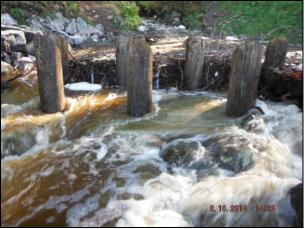
A similar coarse debris trap has also been constructed on the Tower Burn at Rowan Grove. The coarse debris traps consist of wooden poles projecting from a concrete base which will catch coarse debris such as tree trunks and branches that may cause blockages in culverts downstream. This will help reduce potential flooding.
