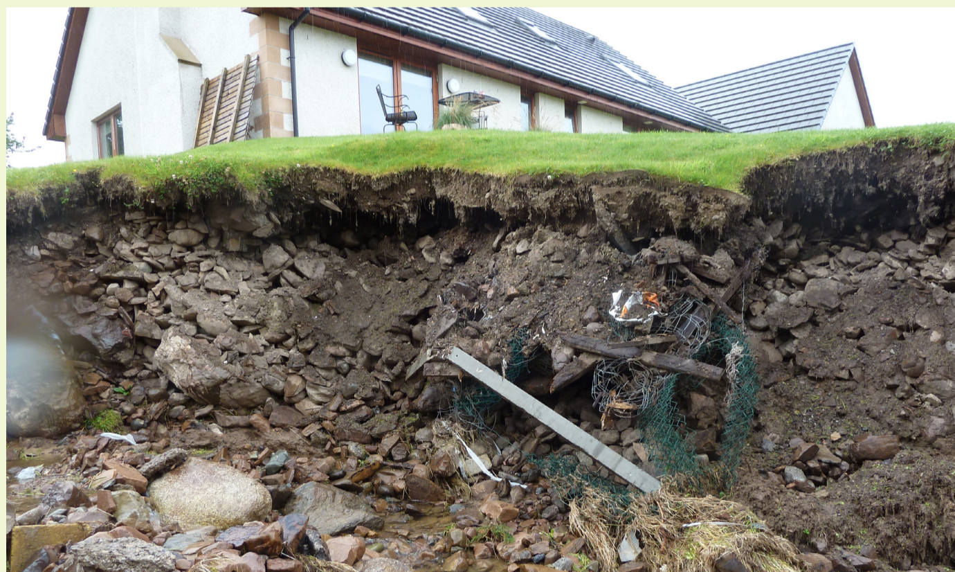
Smithton Burn, upstream of Woodside Village Road
