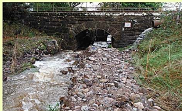
Coarse sediment deposition upstream of the railway at Murray Terrace
