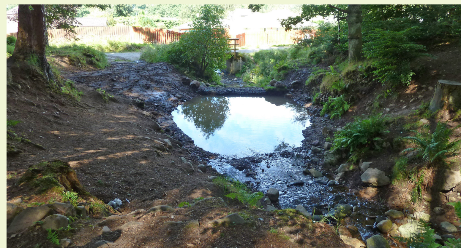
Before: silt trap in Culloden Woods. Silt traps starve downstream channels of sustainable sediments and encourage further erosion downstream.
