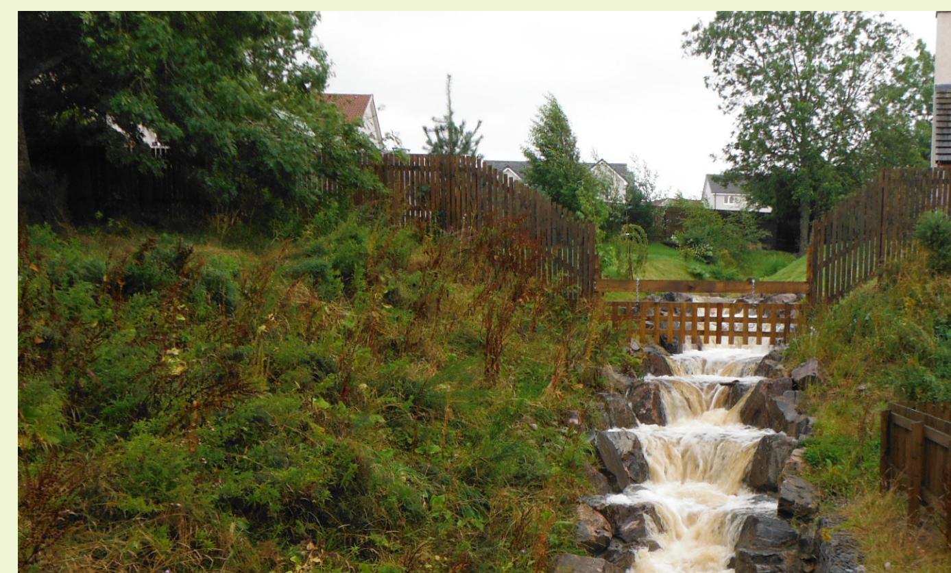
After: newly constructed step pools that dissipate flow energy and are erosion resistant
