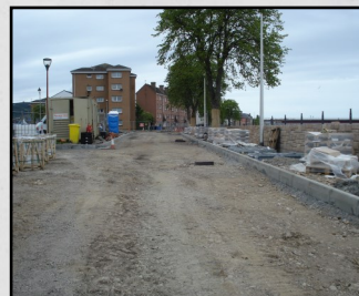
Surface Reinstatement Preparation Huntly Place/Gilbert Street
