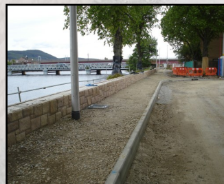
Surface Reinstatement Preparation Riverside Street
