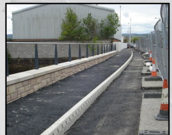
Drainage Kerbing & Surface Reinstatement Kessock Road
