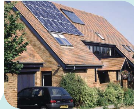
An example of solar PV on a home
