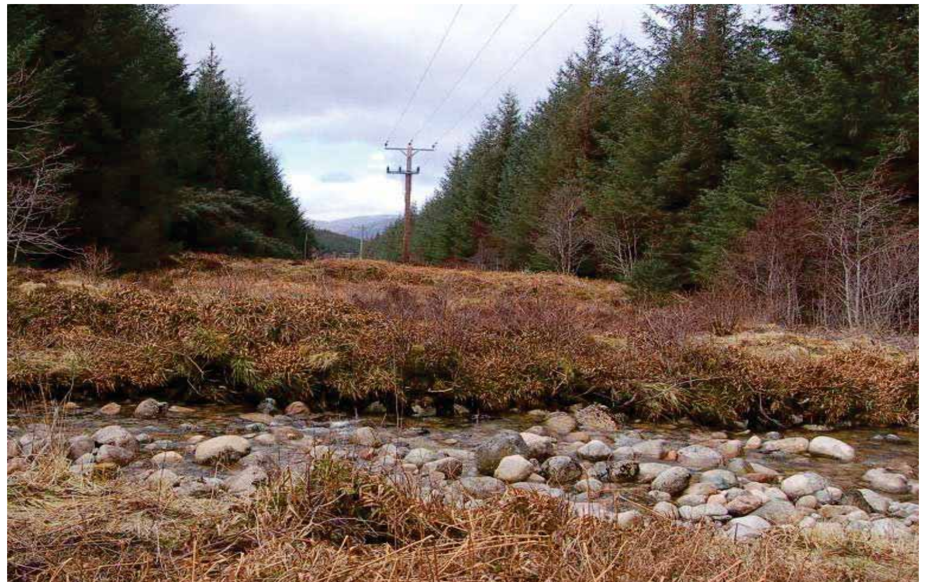
Pylon Line serving Nevis Centre
