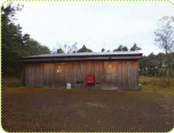
Battery inverter shed
