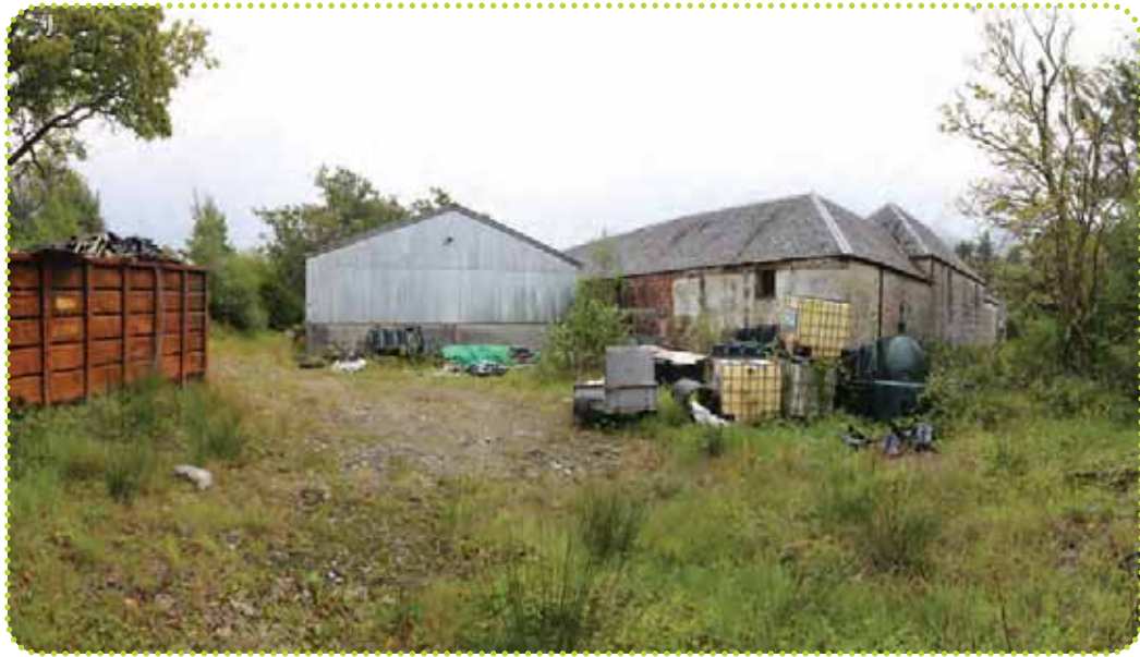
Byre and mechanics shed
