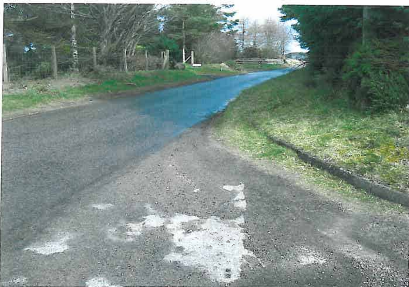
Photo 8 - Existing Site Access View From 2.4m Visibility Point looking East (right)
