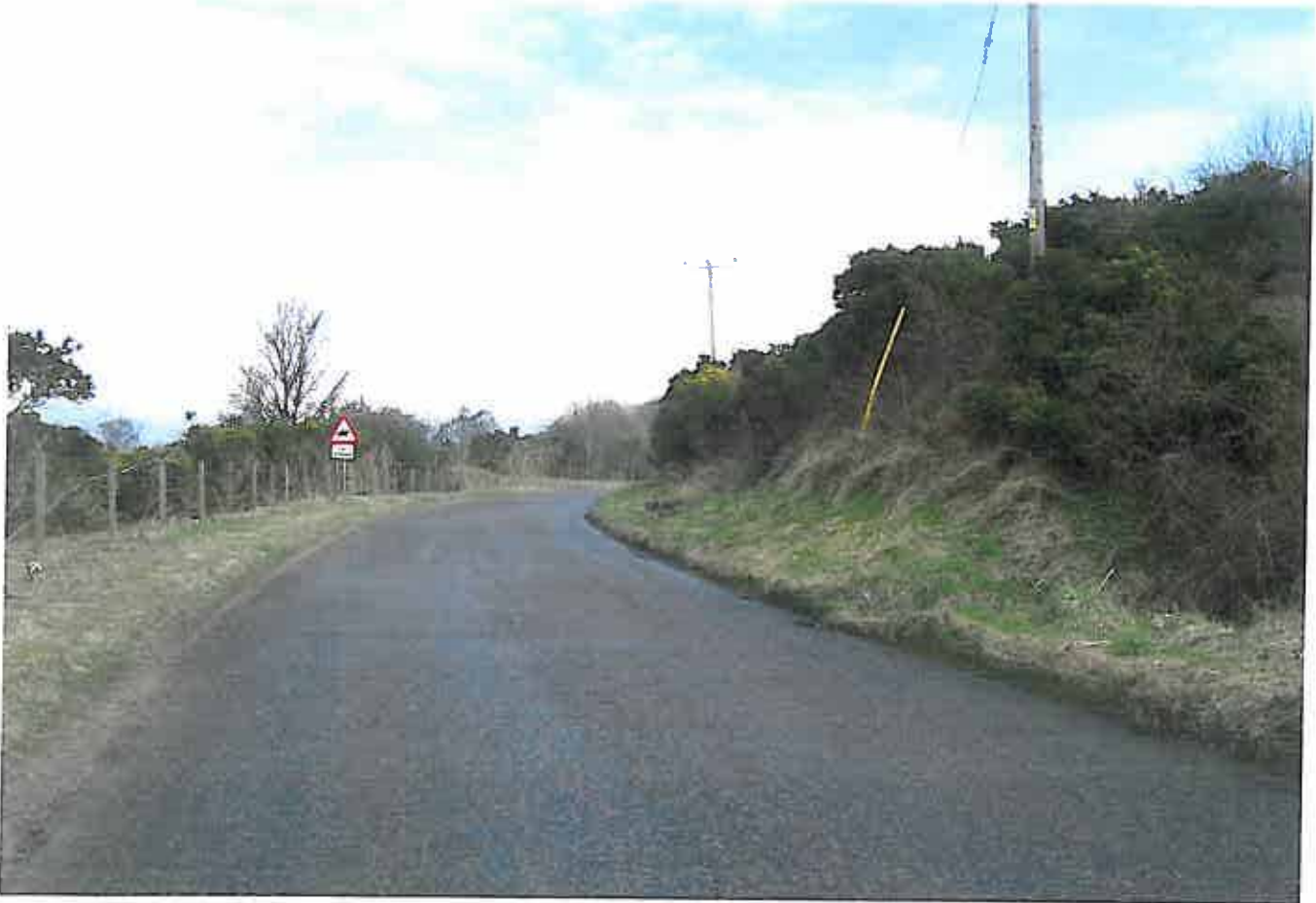
Photo 4 - Restricted Visibility Location 2, looking East
