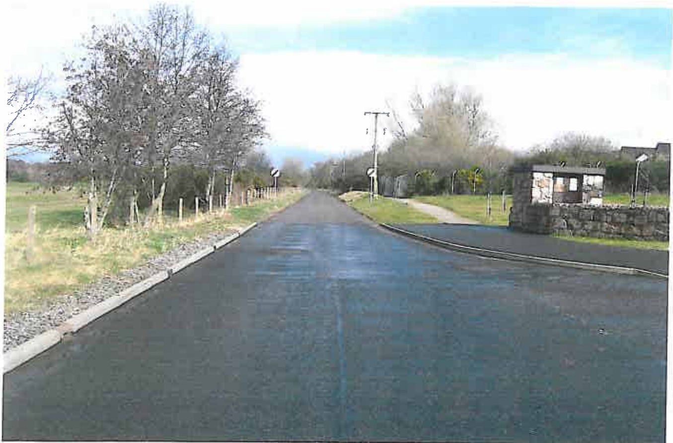
Photo 2 - Looking East on Lochloy Road from Montomerie Drive junction where road width reduces from 6.0m to between 4.7 and 5.0m
