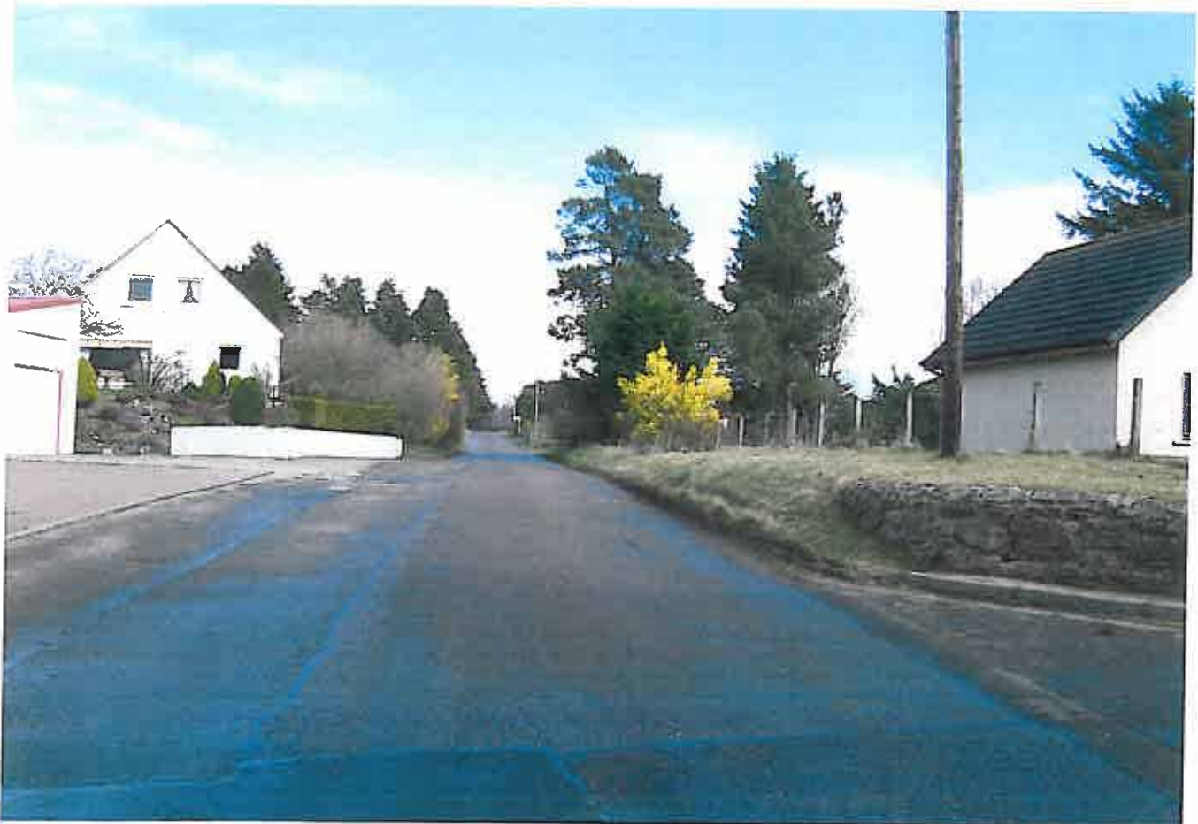
Photo 6 - View looking East along Lochloy Road from West end of Kingsteps
